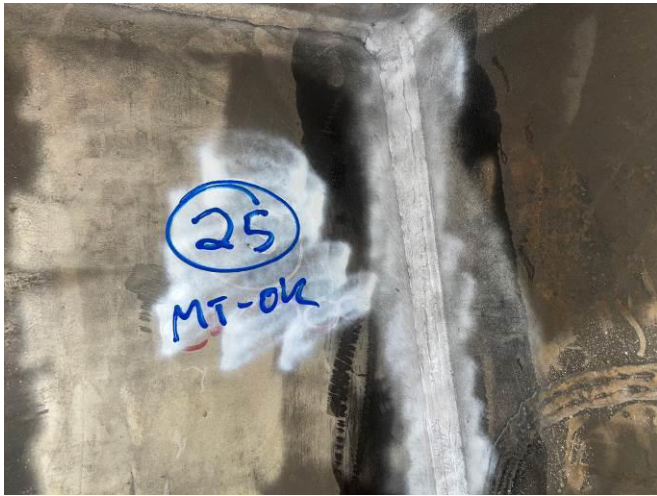
PHOTOGRAPH NO. 74 - INTERNAL BAY ‘C’ TYPICAL VIEW OF REPAIRED DEFECT #27
