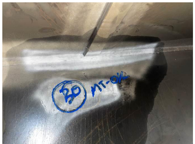
PHOTOGRAPH NO. 77 – INTERNAL BAY ‘C’ TYPICAL VIEW OF REPAIRED DEFECT #30
