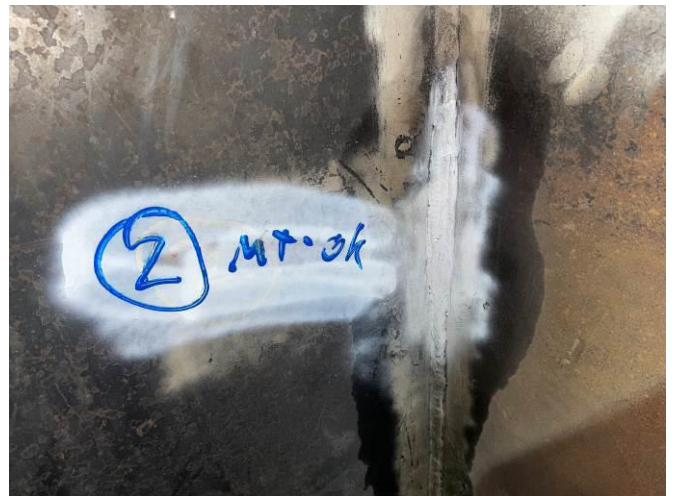
PHOTOGRAPH NO. 51 – INTERNAL BAY ‘C’ TYPICAL VIEW OF REPAIRED DEFECT #4
