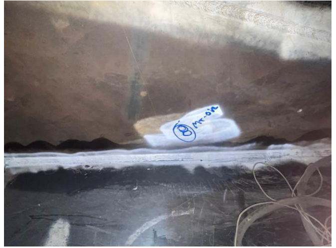
PHOTOGRAPH NO. 57 – INTERNAL BAY ‘C’ TYPICAL VIEW OF REPAIRED DEFECT #10
