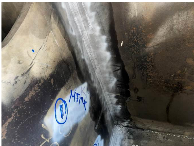
PHOTOGRAPH NO. 58 – INTERNAL BAY ‘C’ TYPICAL VIEW OF REPAIRED DEFECT #11
