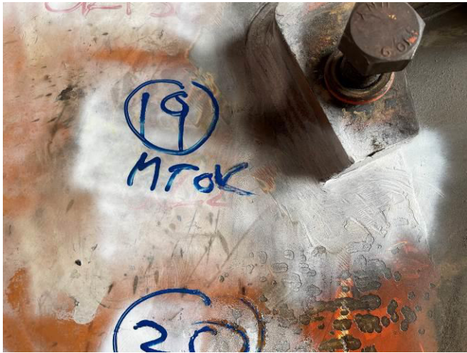
PHOTOGRAPH NO. 21 – EXTERNAL STICK TYPICAL VIEW OF REPAIRED DEFECT #21
