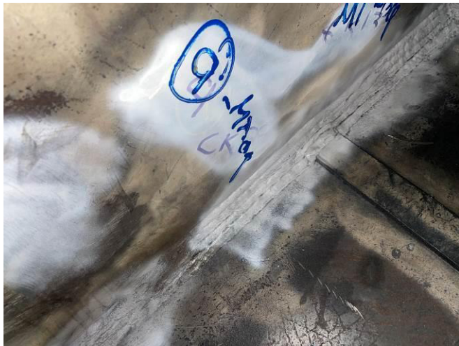
PHOTOGRAPH NO. 58 – INTERNAL BAY ‘C’ TYPICAL VIEW OF REPAIRED DEFECT #11
