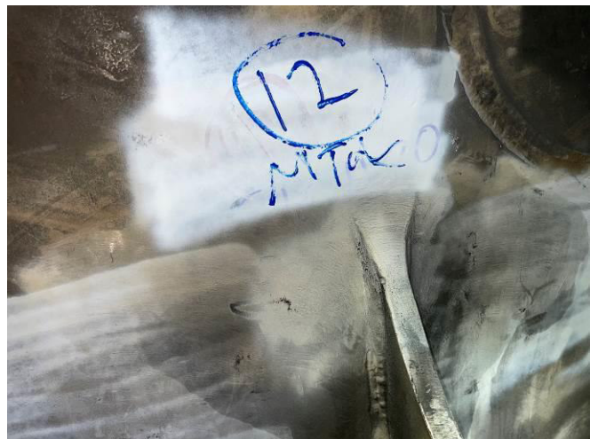
PHOTOGRAPH NO. 59 – INTERNAL BAY ‘C’ TYPICAL VIEW OF REPAIRED DEFECT #12
