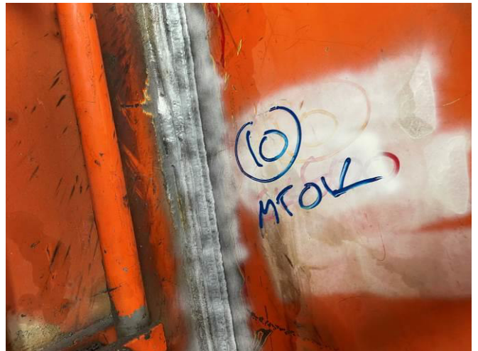
PHOTOGRAPH NO. 12 – EXTERNAL STICK TYPICAL VIEW OF REPAIRED DEFECT #12
