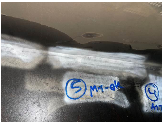
PHOTOGRAPH NO. 52 – INTERNAL BAY ‘C’ TYPICAL VIEW OF REPAIRED DEFECT #5
