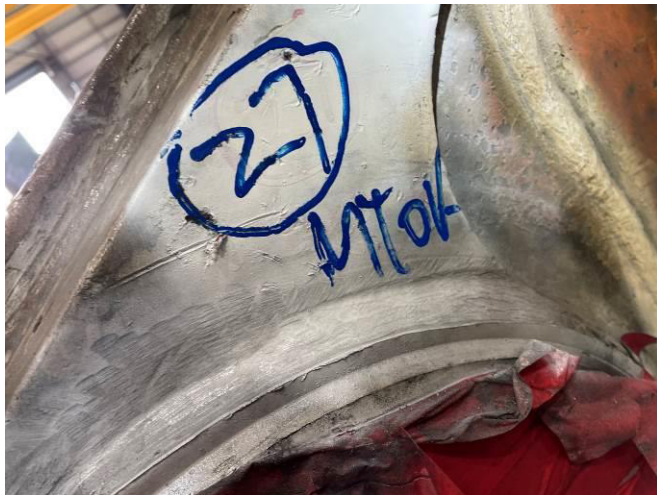
PHOTOGRAPH NO. 29 – EXTERNAL STICK TYPICAL VIEW OF REPAIRED DEFECT #29
