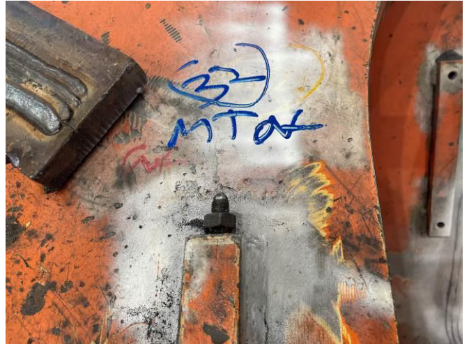
PHOTOGRAPH NO. 34 – EXTERNAL STICK TYPICAL VIEW OF REPAIRED DEFECT #34
