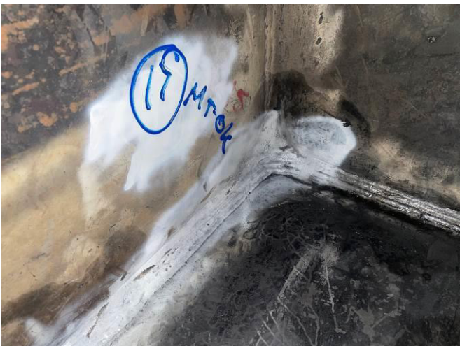
PHOTOGRAPH NO. 64 – INTERNAL BAY ‘C’ TYPICAL VIEW OF REPAIRED DEFECT #17
