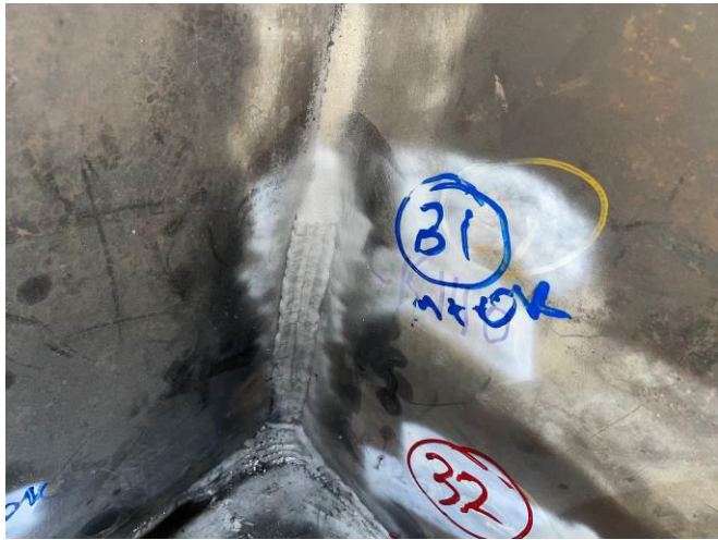
PHOTOGRAPH NO. 80 - INTERNAL BAY ‘C’ TYPICAL VIEW OF REPAIRED DEFECT #33
