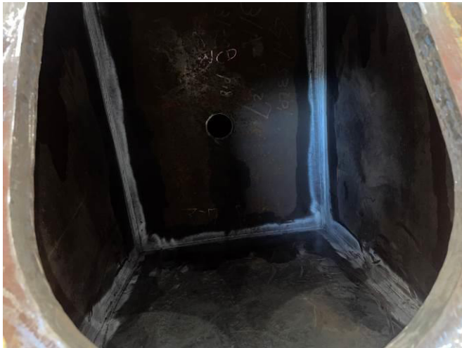
PHOTOGRAPH NO. 6 – GENERAL VIEW OF INTERNAL BAY ‘A’
