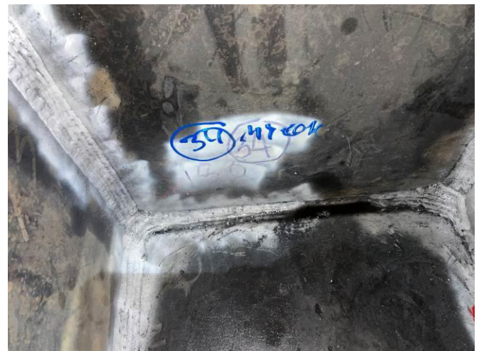
PHOTOGRAPH NO. 81 – INTERNAL BAY ‘C’ TYPICAL VIEW OF REPAIRED DEFECT #34
